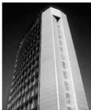
Burda Hochhaus, Offenburg
