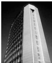
Burda Hochhaus, Offenburg
